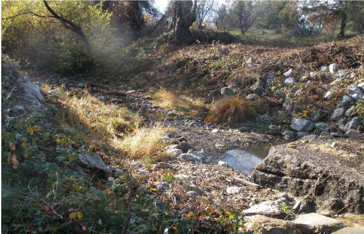
PHOTOGRAPH 7 Crowley Gulch Downstream of Well No. 2 Study Area, View South
